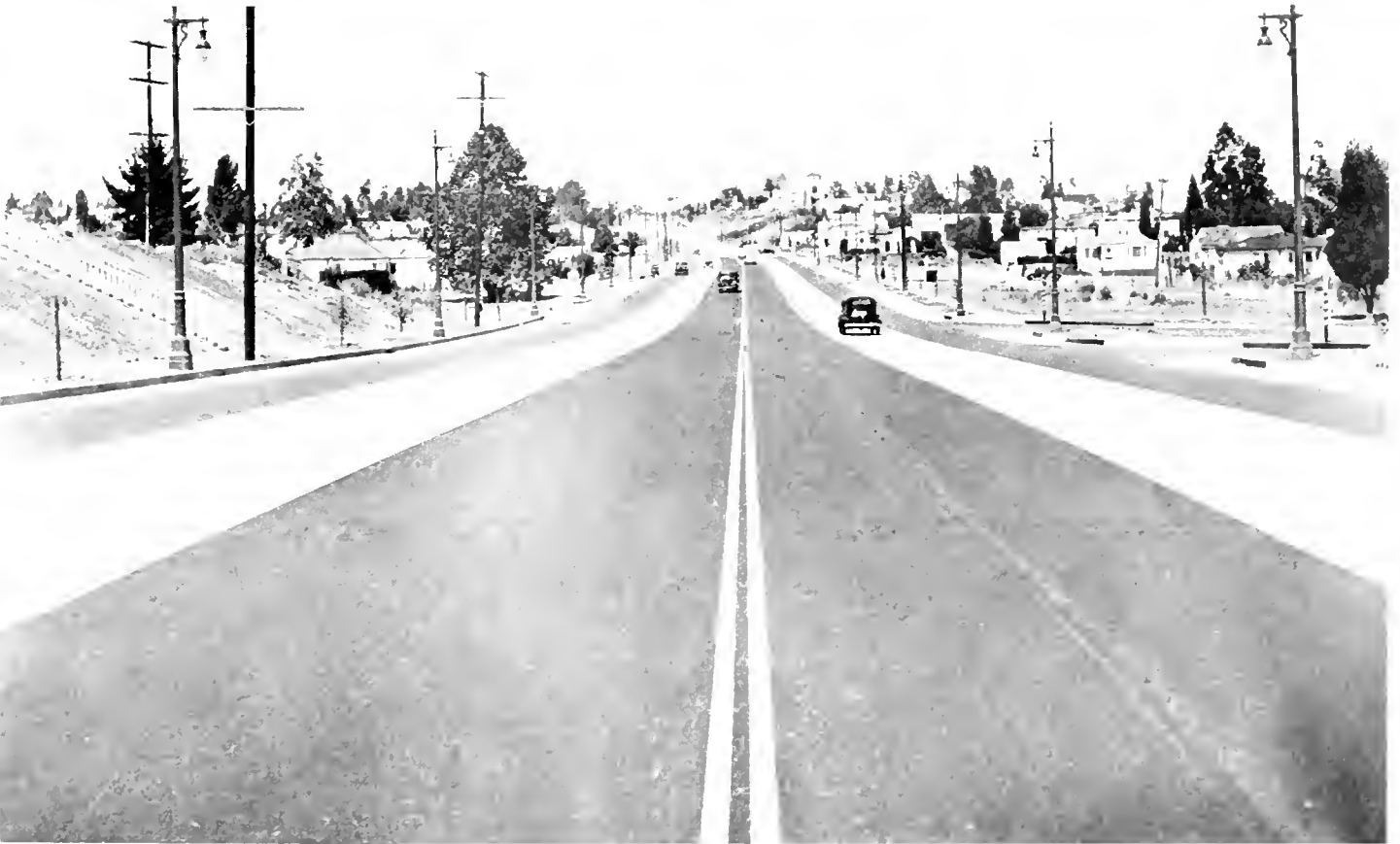
This Olympic Boulevard unit has 4 twelve-foot lanes of asphaltic concrete, 2 eleven-foot lanes of Portland cement concrete
